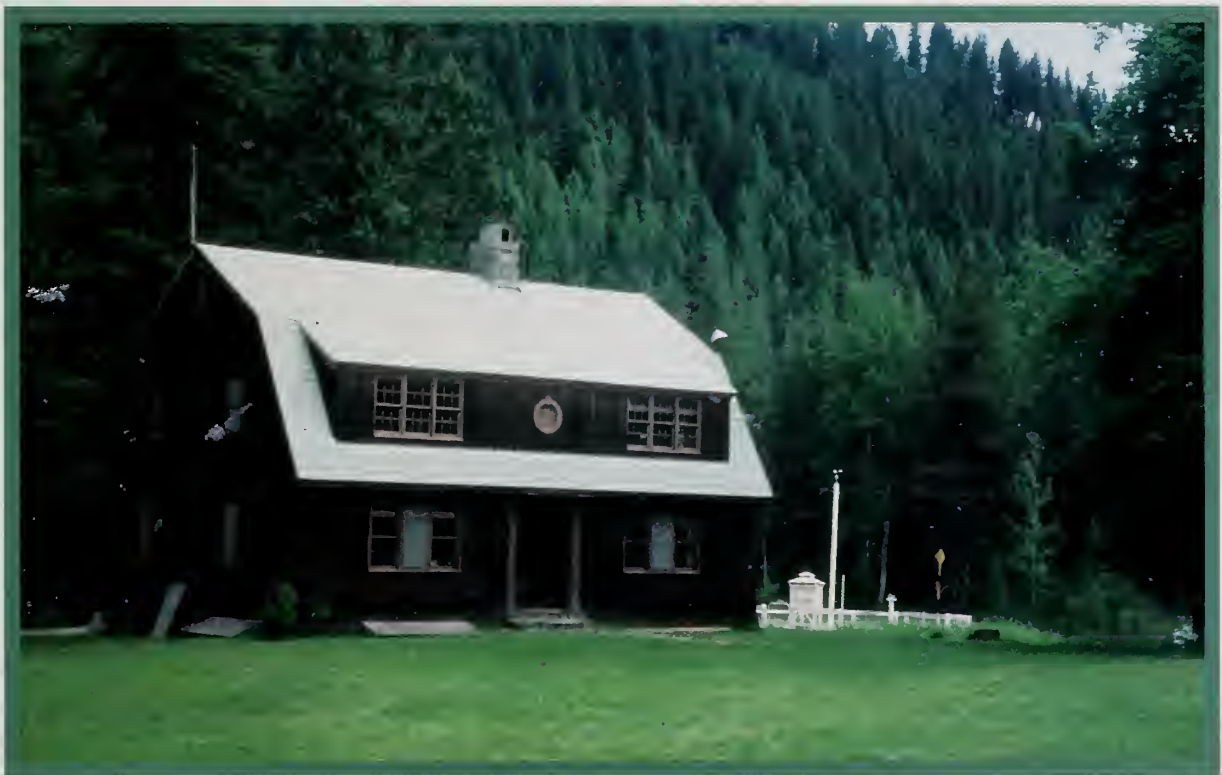
Headquarters building at Priest River Experimental Forest.
